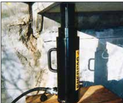
◀ The portable lock nut cylinder RACL-1506 used for extended load supports during epoxy injection for bridge reinforcement.
