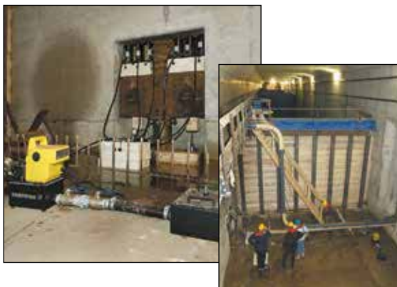
◀ The unique Enerpac RA-Series cylinders – lightweight and entirely made of aluminium alloy – these RAC-506 cylinders are ideal for the positioning of tunnel elements under the river. (High Speed Train Line, The Netherlands)
