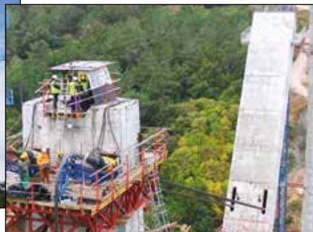
▼ Two concrete arches of this viaduct in Silleda, Spain are rotated and lowered by Enerpac Heavy Lifting Strand Jacking Systems.
